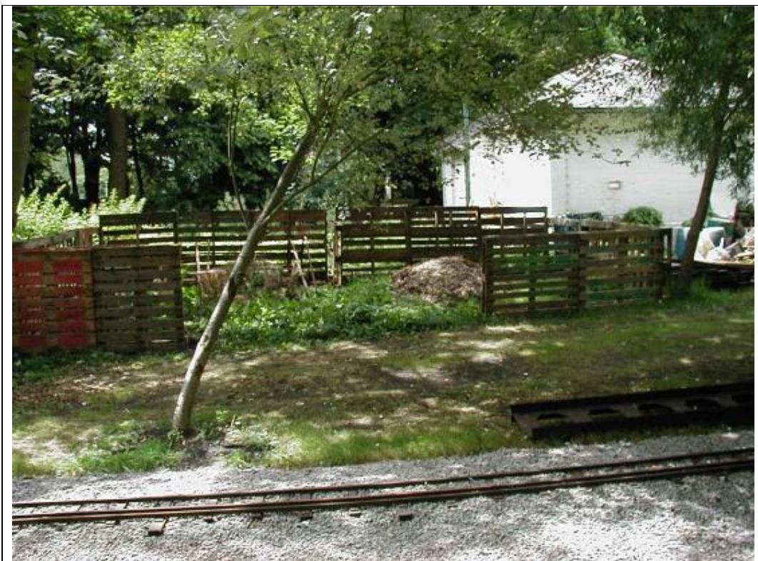
The new compost bin is constructed
