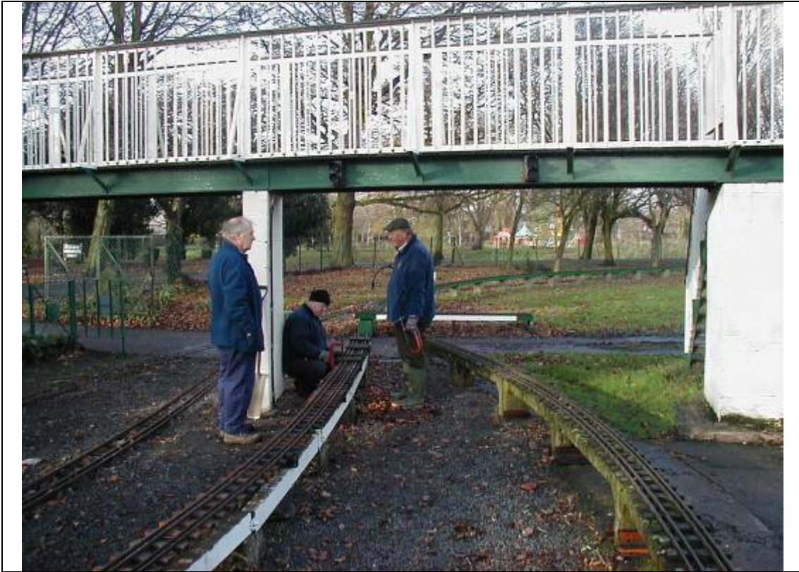
New sleepers are fitted to the raised track
