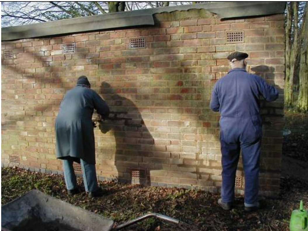
Roy and Dick re-point the opposite side of the building
