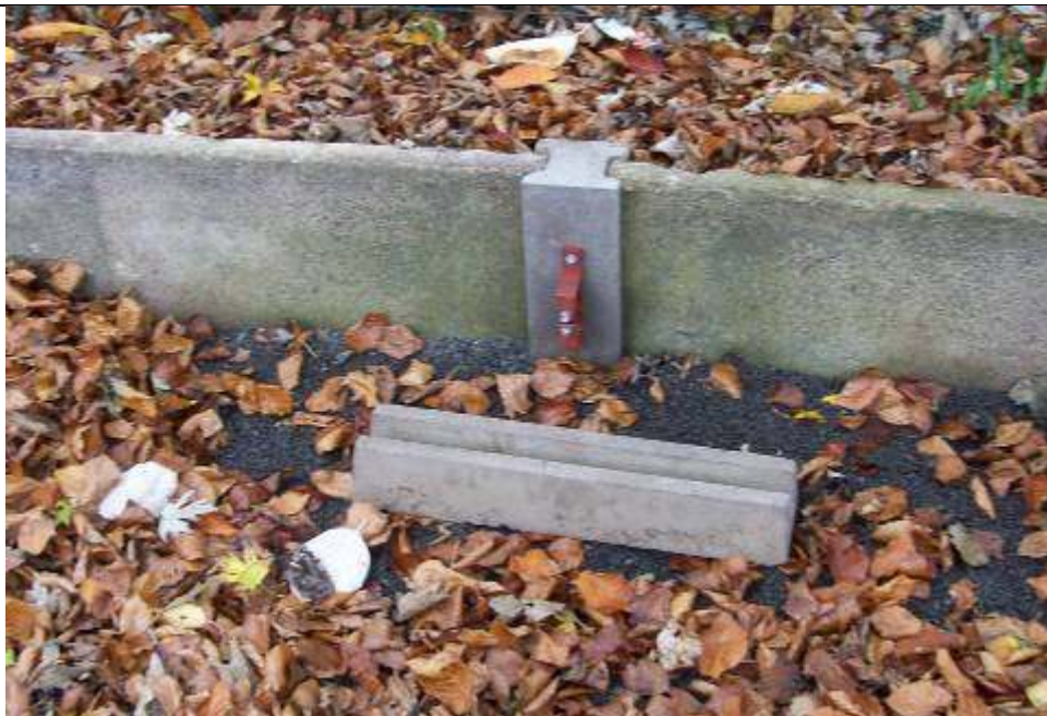
Point rods to control the station points are starting to come together.
