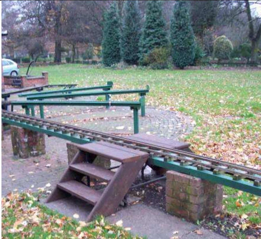
The new steps over the steaming bay access track are complete
