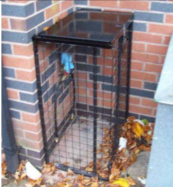
The gas bottles that will be stored outside has had a lockable cage built so they remain secure.
